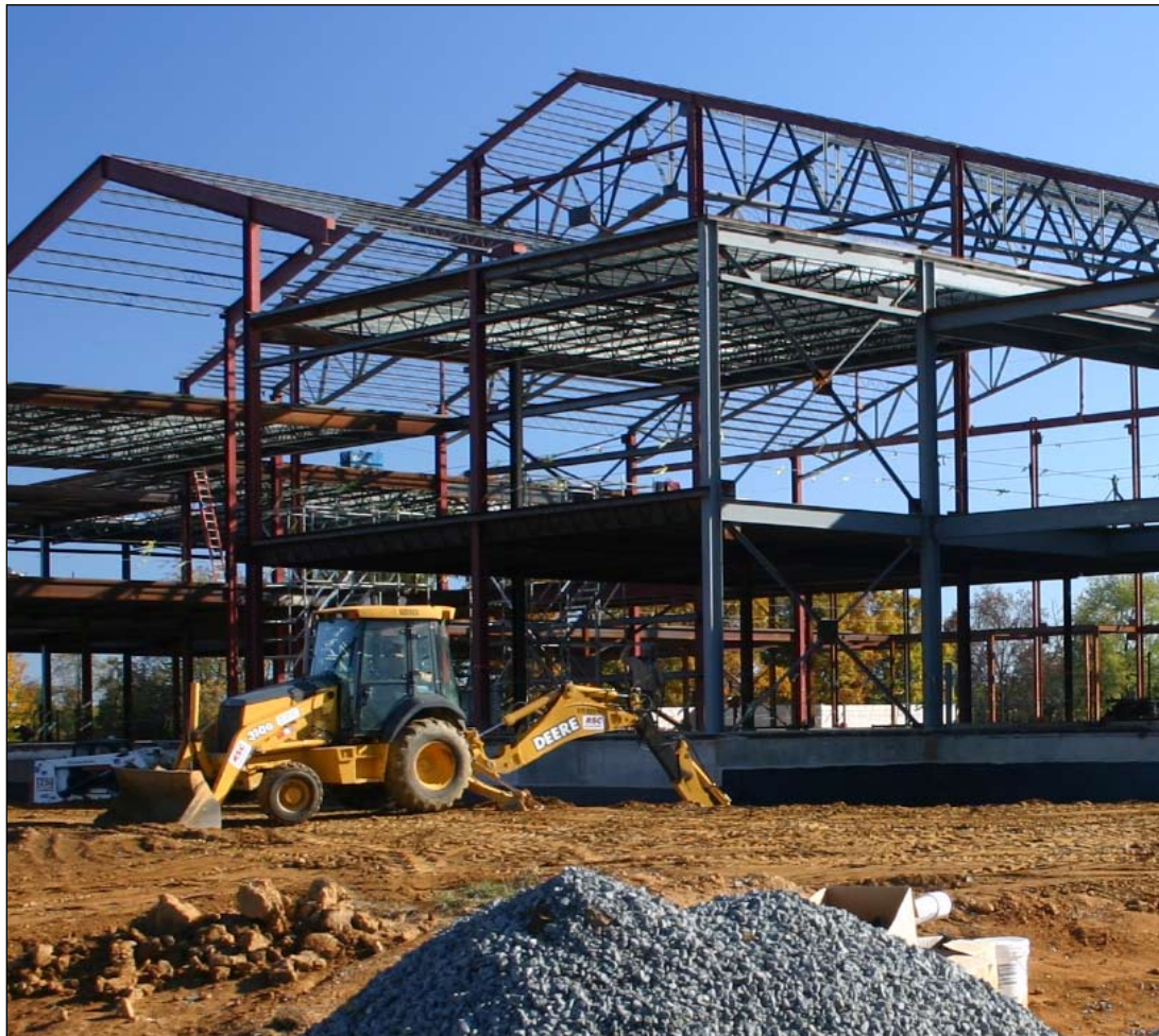
The Barbara Hodel Center, under construction at Patrick Henry College.
